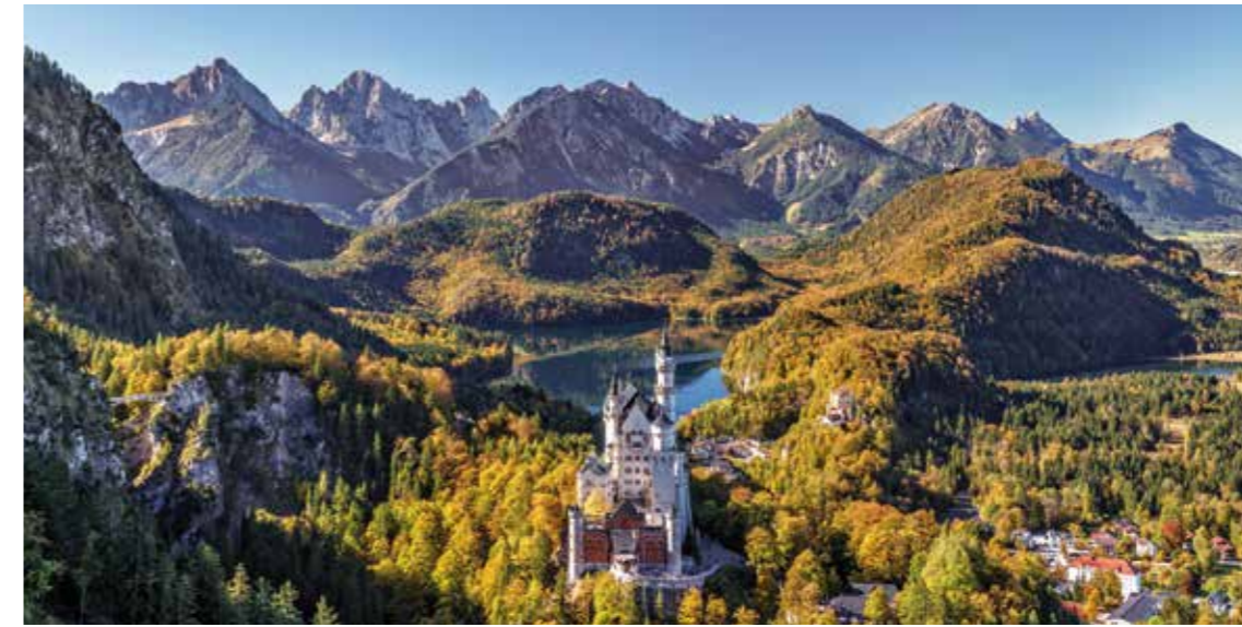
Neuschwanstein Castle: The facade was treated with silicone resin emulsion paints based on WACKER products, ensuring that subsequent generations will be able to enjoy all of its splendor.
