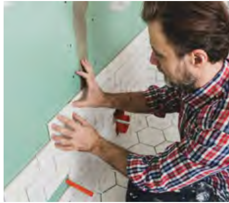
When tile adhesives are installed on dry walls, a primer is required prior to the laying of the tiles. A flexible tile adhesive best copes with movements of the dry wall. This, together with a hydrophobic grout mortar, is important.
