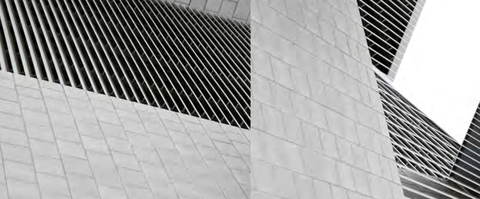
Tiles are applied on facades
