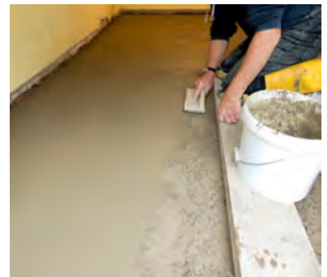
Surfaces with undulations and irregularities increase the likelihood of a tiling failure, in addition to an imperfect surface level. In this case, the use of a self-leveling flooring screed can be quite beneficial, as it offers the tiler a smooth and even surface to lay the tiles on in the case of a flooring application.
