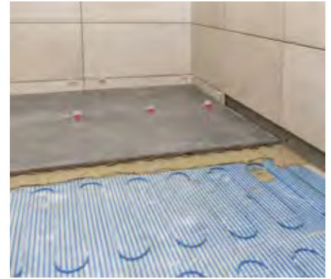
Floor heating is especially demanding. Highly flexible tile adhesives are necessary to compensate stresses resulting from different heat expansion coefficients of the different layers.
