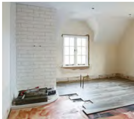
When tiles are installed on wooden subfloors or “old” wooden floors, the tile adhesive must be extremely flexible with a very high adhesive bond strength.
