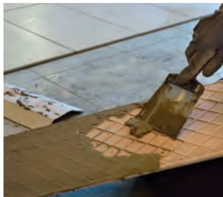
In renovation processes it can be easier and more economical to just lay tiles over tiles. This is possible when polymer-modified tile adhesives are chosen.
