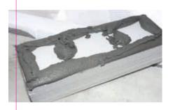
A cementitious, polymer-modified adhesive mortar is required to attach the ETICS to the masonry. It is the dispersible polymer powder in the adhesive mortar that ensures reliable adhesion to both the masonry and the insulation material. Here, the leading binders are WACKER's VINNAPAS® dispersible polymer powders. They are mixed into the dry-mix mortar in the factory, offer reliable processing and guarantee optimum mortar properties.
