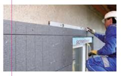
With the right kind of polymers added to enhance the adhesive mortar, external thermal insulation composite systems can be applied to virtually any substrate, e.g.:
