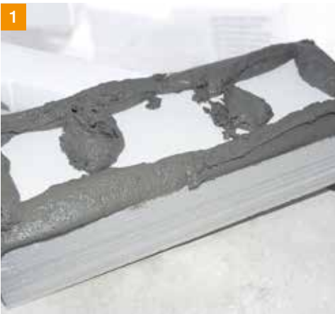
1 Apply adhesive mortar to the thermal insulation panels.
