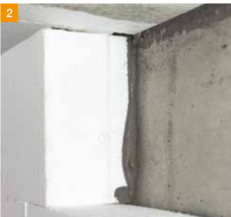
2 Bond the panels to the existing masonry without leaving any joints.
