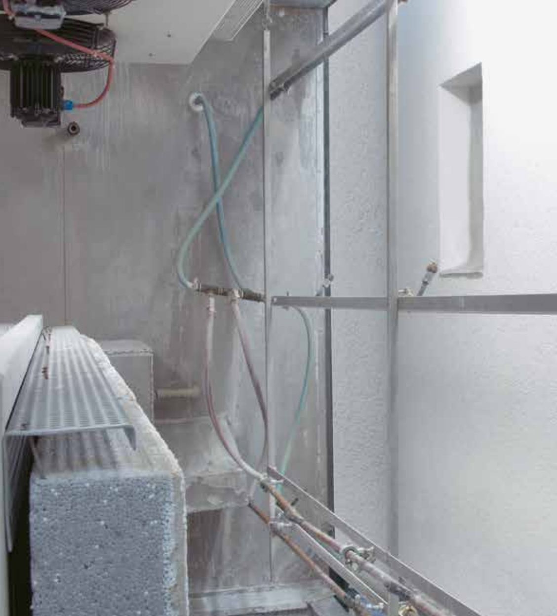
A prepared wall (at right) is sprayed in the EOTA chamber
