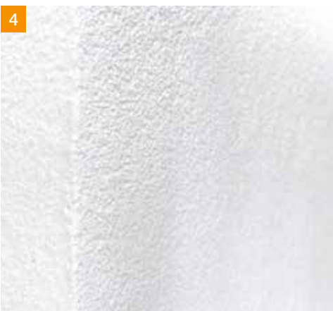
4 Finally, apply a decorative finishing coat to the facade. This coat may be mineral render, synthetic-resin render, silicone render or silicate render, and may be combined with paint.
