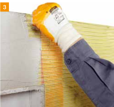
3 After the adhesive has cured, apply the base coat and embed the reinforcing mesh.
