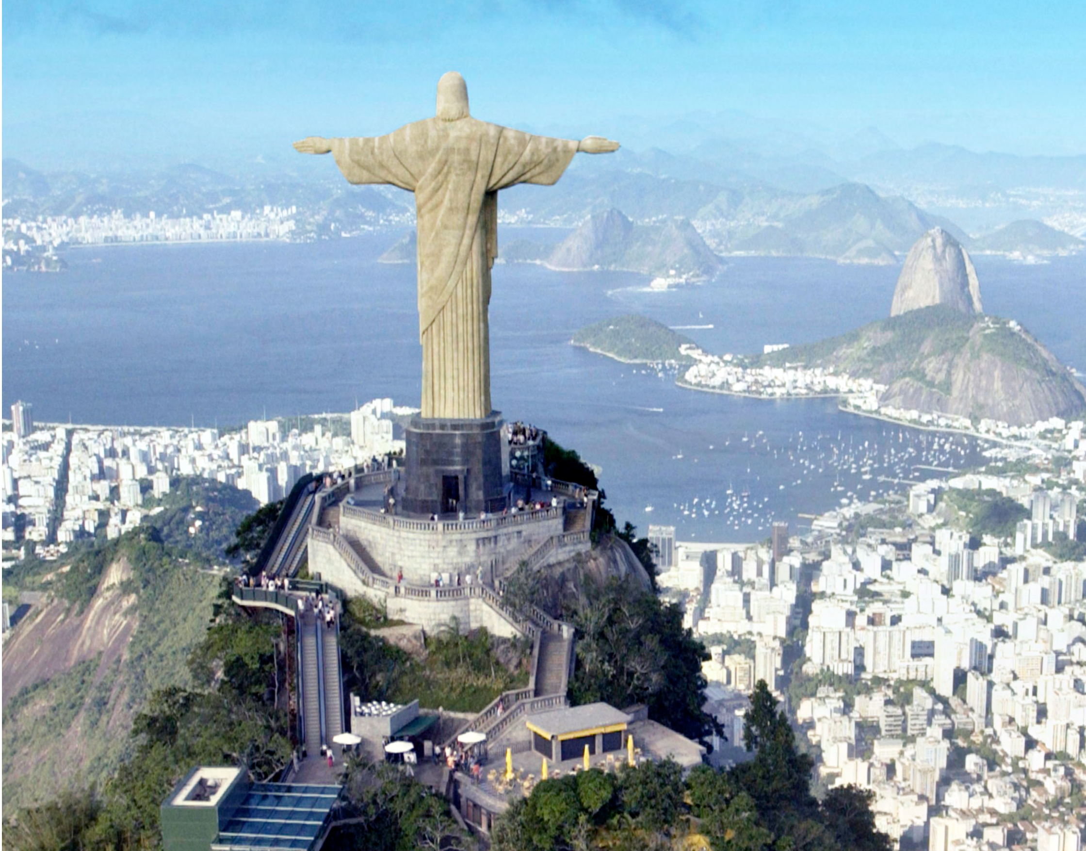
Christ the Redeemer is made of concrete and soapstone: Materials that deteriorate with harmful environmental influences. In 2010, the statue was coated with SILRES® BS 16 to protect and preserve it for the future.
