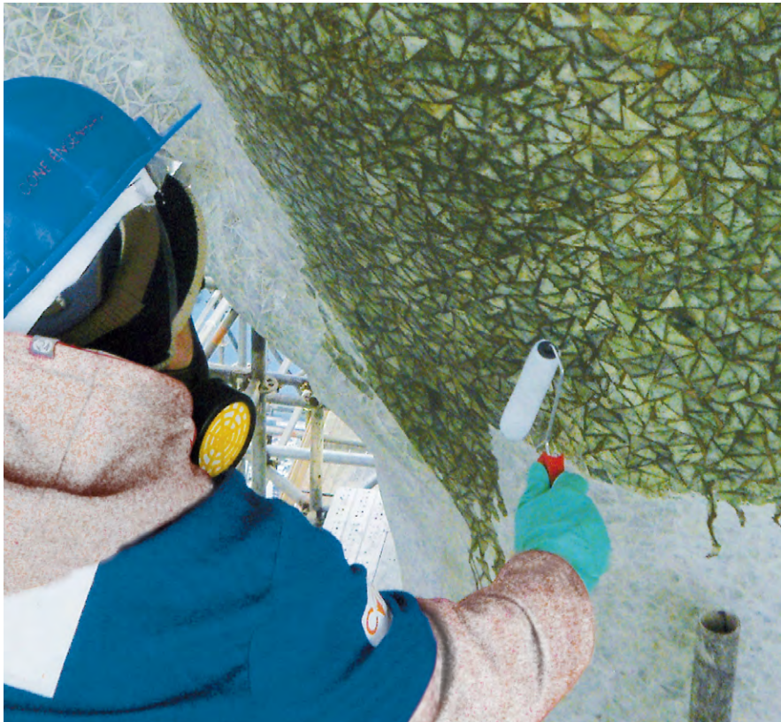
Protection made easy: After the statue was restored for its 80th anniversary, the SILRES® BS 16 solution was simply and efficiently applied to the stone using rollers.
