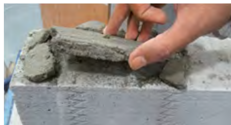
Traditional unmodified mortars show poor adhesion to AAC blocks. The mortar can be pulled off easily.
