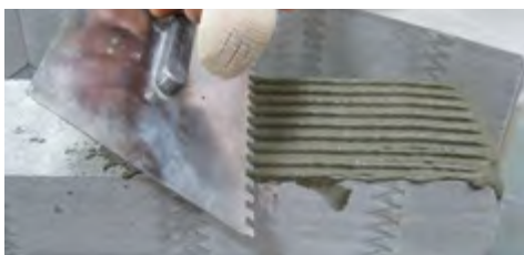
Mortars modified with VINNAPAS® have good wetting properties and can be applied in thin layers of 3 – 5 mm. No prewetting is necessary. This saves material and time.
