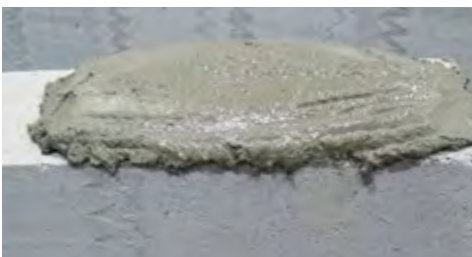
Building with AAC blocks: traditional unmodified mortars have no wetting capability and need to be applied in thick layers of 10 – 20 mm. Plus: the bricks must be prewetted.
