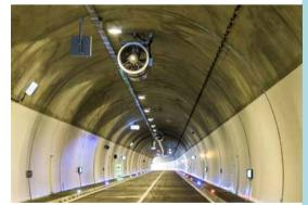
Smoke extractor fans in a road tunnel. In a fire, the fan motors are subject to severe thermal stress. Impregnation with SILRES<sup>®</sup> H60 provides ideal thermal protection.
