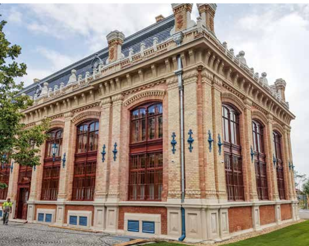
Now restored to its original style: the right wing of the train station with the pavilion that housed the former post office.
