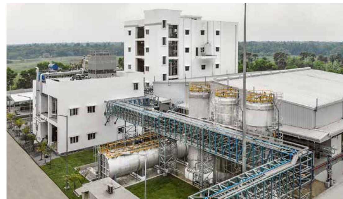
Wacker Metroark Chemicals' new hydrosilylation plant at its Amtala site near Kolkata.
