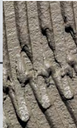
Large-format tiles are on trend, but the tile adhesives used must meet special requirements.
