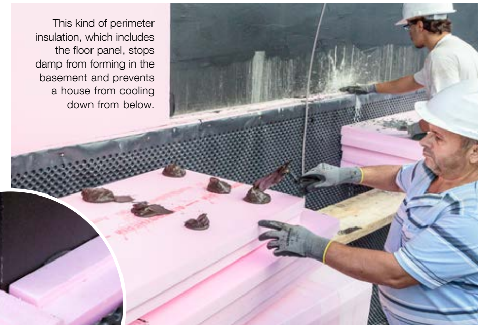
Styrofoam or other foamed plastic insulation panels are placed on the bitumen barrier layer to provide the basement wall with insulation against energy loss.
