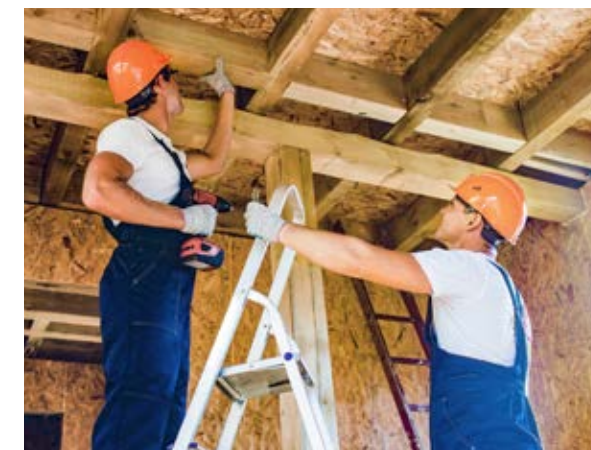
Ants like to build their nests in the roof truss of houses and can cause considerable damage to the beams and insulation.
