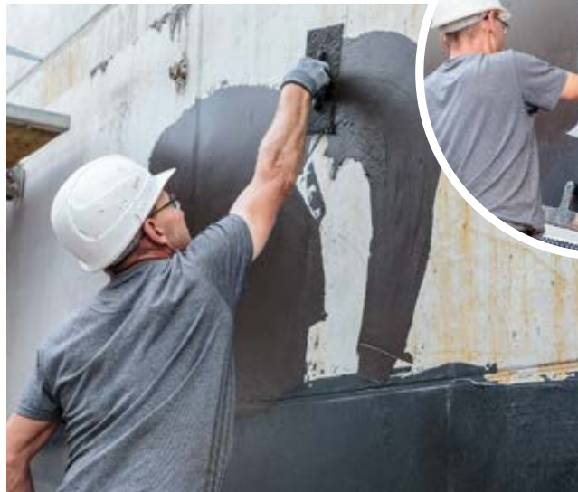
Builders use polymer-modified bitumen to seal basement walls watertight.
