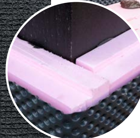
Styrofoam or other foamed plastic insulation panels are placed on the bitumen barrier layer to provide the basement wall with insulation against energy loss.
