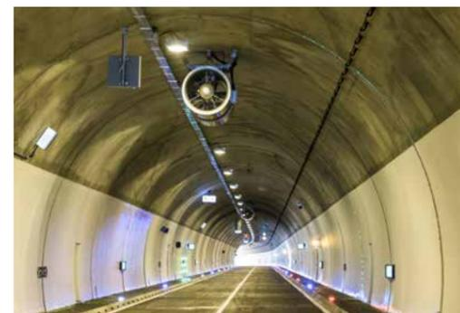
Smoke extractor fans in a road tunnel. In a fire, the fan motors are subject to severe thermal stress. Impregnation with SILRES® H60 provides ideal thermal protection.
