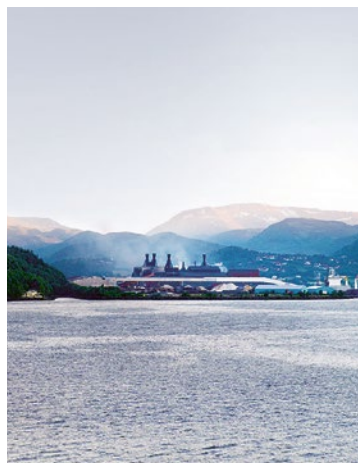
Silicon-metal production site in Holla, Norway
