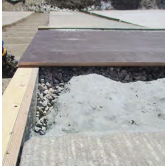
The self filling concrete is applied.
