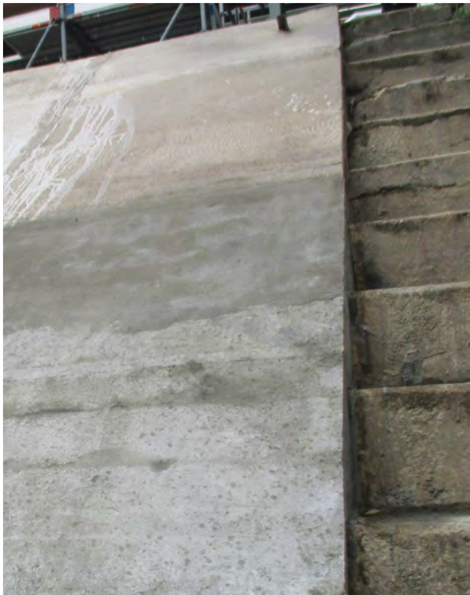
After: A smooth, crack-free surface. The repair was made using self-filling concrete including ETONIS®.
