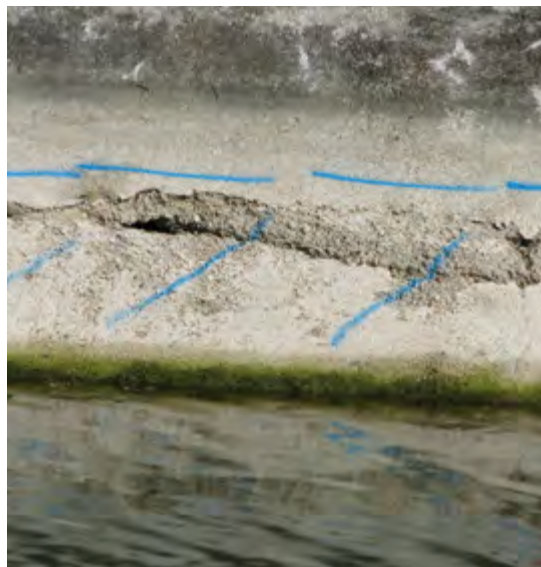
Although the old concrete was still in good condition, there was damage to the canal in many areas.
