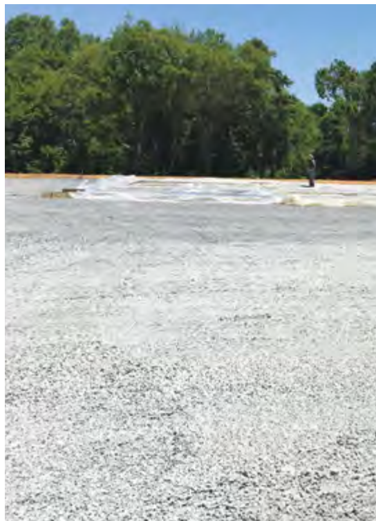
Researchers install the modified pervious concrete
