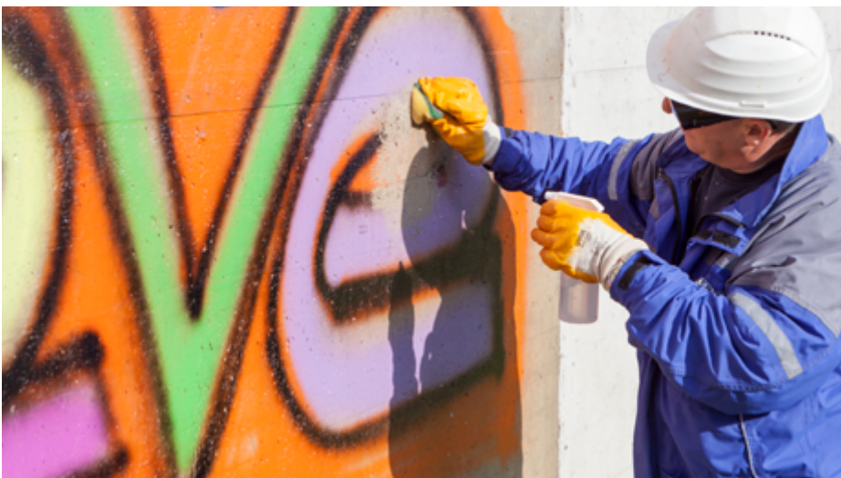
Removal of graffiti: Poor adhesion of graffiti paints on surfaces treated with SILRES® BS 710. Paints can be removed easily with a wet tissue or sponge.
