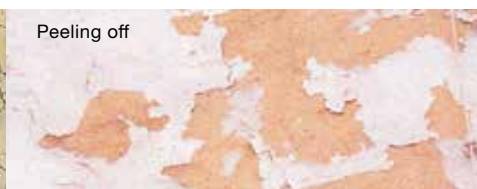
Salt efflorescence
