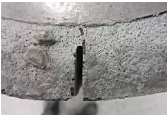
Figure 4: Cut into the concrete ring, without stress release cracking. SFCC during demolding from the ASTM C 1581 ring after 96 d of testing. No substantial crack appeared.
