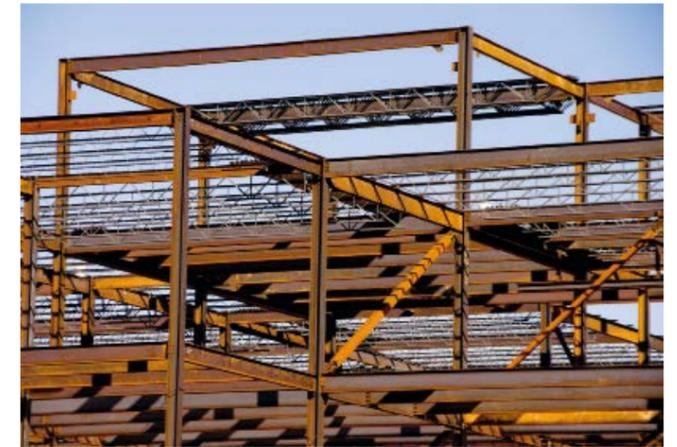
Thanks to prefabricated parts and bolted joints, steel frames can be assembled quickly and easily – thereby providing ideal construction of storage depots, for example.
