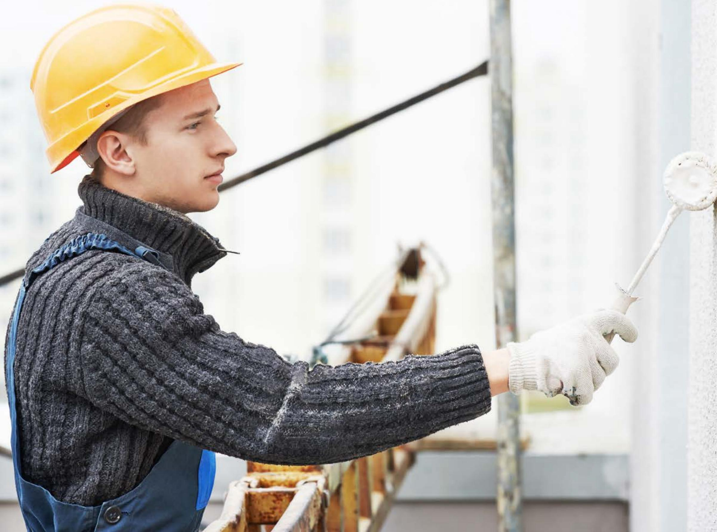
Paints and plasters generally only set adequately if the temperature remains above 5°C for several days. Otherwise the waterborne systems will freeze. PRIMIS® KT 3000 shortens the setting time substantially.
