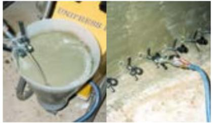
4. Inject cement slurry in the case of cracked masonry.
