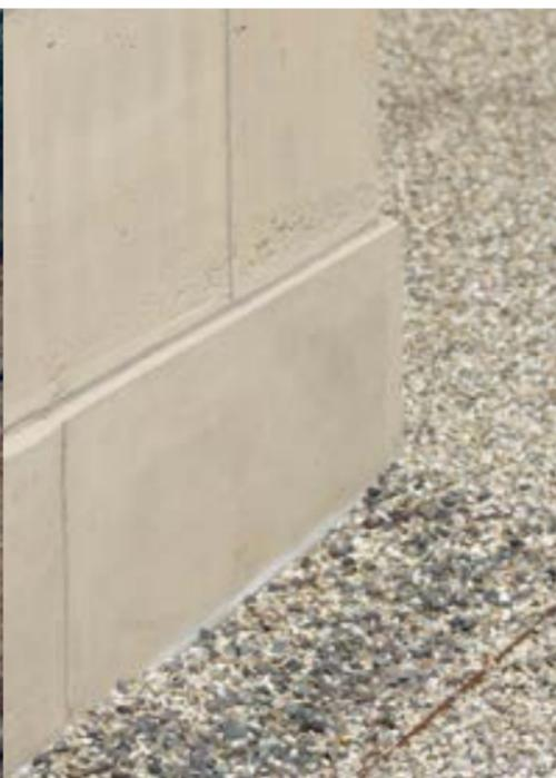
Close-up of a Bugatti Palace exterior wall after restoration with SILRES® BS.
