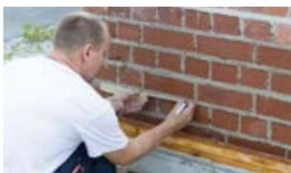
1. Mark the distance between the holes and determine the drilling depth.
