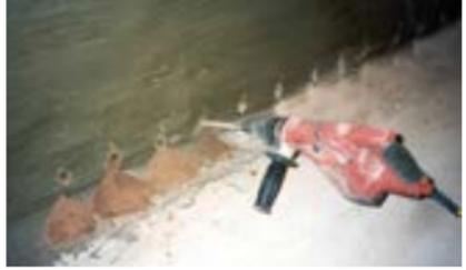
2. Mark the distance between the holes and drill them, then blow out drilling dust.
