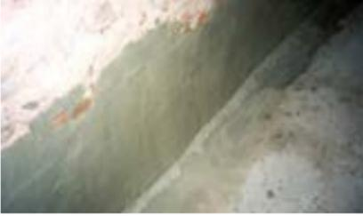
1. Level the surface, apply sealing slurry and determine the drilling depth.
