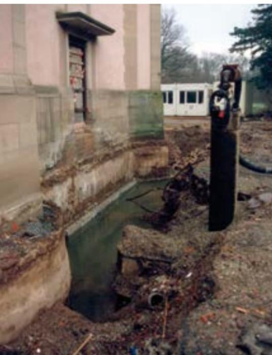
Example of moisture damage: the Bugatti Palace in Molsheim (Alsace, France) displayed severe damage due to groundwater prior to its renovation in 2000.
