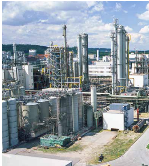
A new silane distillation column went into operation in 2022. It is not only higher than its 1972 counterpart, but also more effective and energy-efficient.
