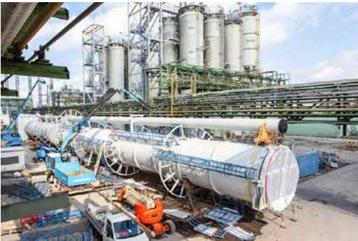
A new silane distillation column went into operation in 2022. It is not only higher than its 1972 counterpart, but also more effective and energy-efficient.
