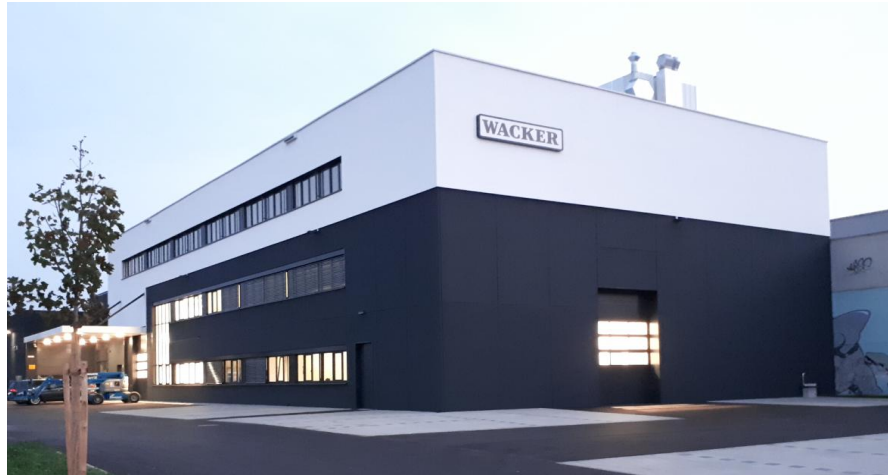
Innovation hub Lindach, BGH Germany
