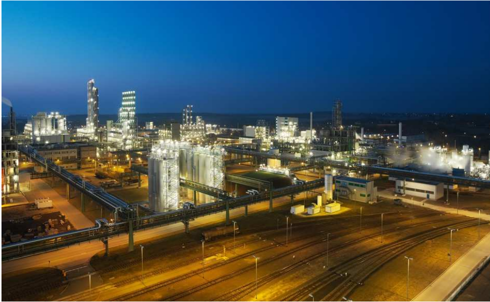
WACKER manufactures silicones and polysilicon at its site in Nünchritz, Germany. In 2022, the chemical company will also start producing hybrid polymers for adhesives and sealants at the plant. (Photo: WACKER)
