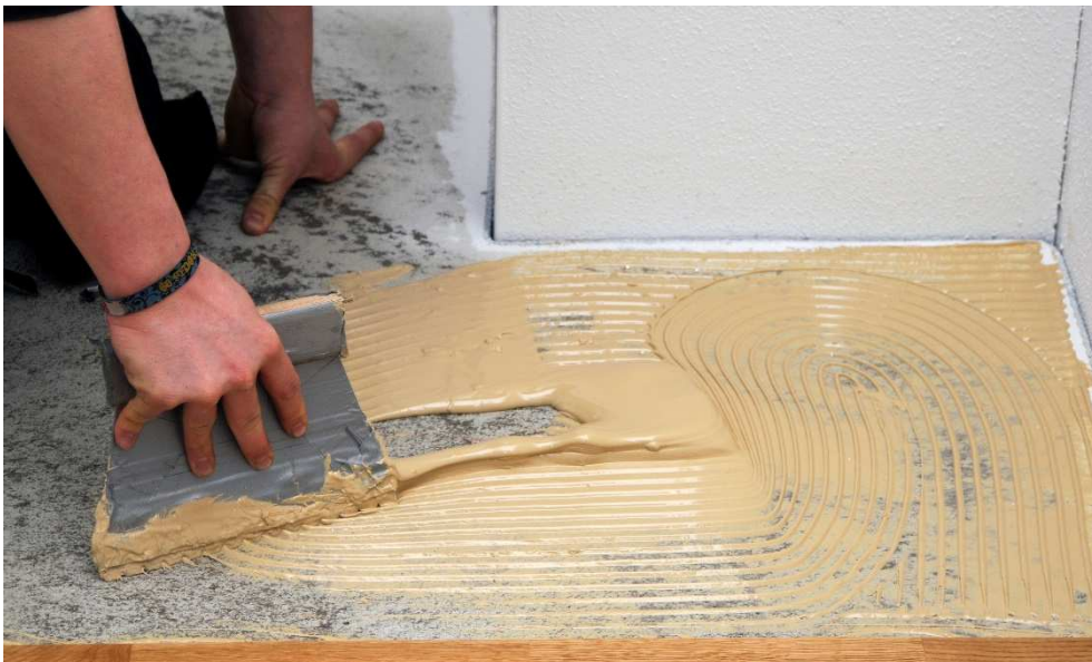
Wood-flooring adhesives formulated with GENIOSIL® adhere well, are highly elastic and have a low environmental impact, because they are solvent-free. (Photo: WACKER)
