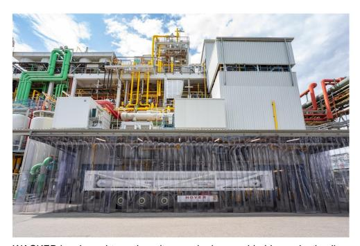
WACKER has brought another ultrapure hydrogen chloride production line on stream at its Burghausen site in Germany. The chemical is an important processing aid for the semiconductor industry. (Photo: WACKER)
