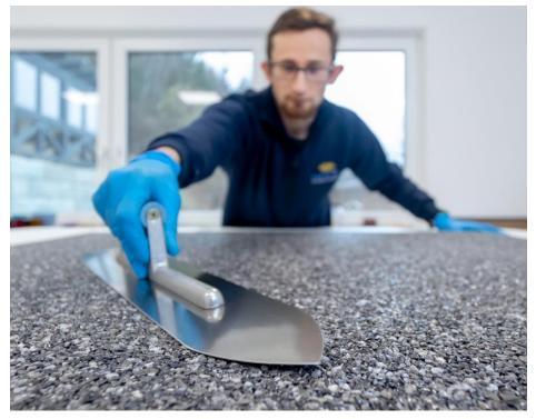
The silicone resin SILRES® BS 6920 can be used to produce resin systems for fixing floor coverings made of stone granules. WACKER will be unveiling the product at the 2023 European Coatings Show in Nuremberg. (Photo: WACKER)
