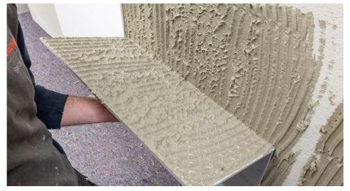
VINNAPAS® 4419 E and VINNAPAS® 8819 E are polymeric binders that improve the wetting properties of tile adhesives, allowing for long correction times. WACKER will be presenting the new products at ECS 2023. (photo: WACKER)
