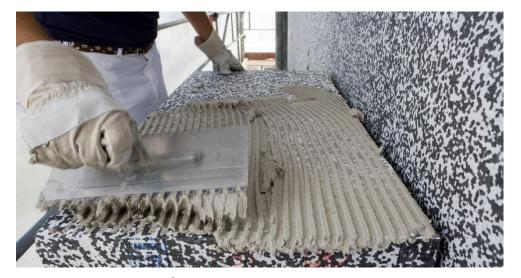
WACKER's VINNAPAS® 4449 E polymeric binder was developed especially for formulating adhesive mortars for exterior insulation and finish systems (EIFS). Benefits of the product include its ability to form exceptionally strong bonds within the layer system and perfectly balance the forces that arise as a result of temperature fluctuations and other influences. WACKER will be unveiling the product at ECS 2023 in Nuremberg. (photo: WACKER)
