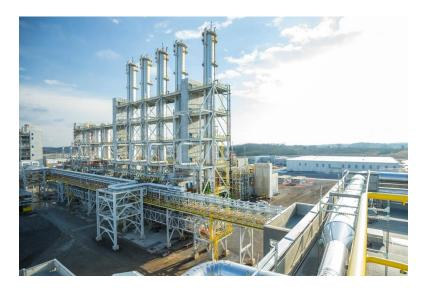
Distillation columns for the production of trichlorosilane at the Charleston site in the U.S. state of Tennessee. WACKER has been producing high-purity polysilicon there since 2015, and HDK® brand pyrogenic silica since 2019.
