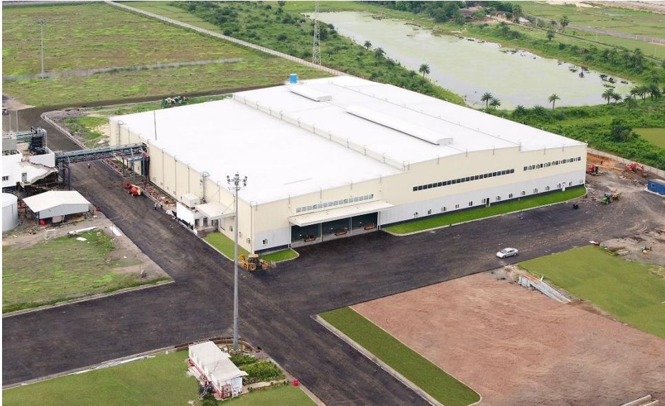
Areal view of the new production site in Panagarh, India. Production currently includes solid and liquid silicone elastomers as well as ready-to-use silicone compounds. (photo: WACKER)
