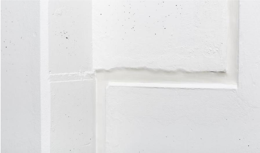
GENIOSIL® XM 25, a gamma-silane-terminated polyether, allows the formulation of low-modulus sealants with exceptionally high elastic recovery. Potential applications include sealants for expansion joints in buildings made of industrially prefabricated concrete parts (photo: Wacker Chemie AG)
