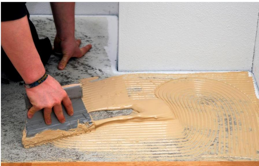
At the European Coatings Show, WACKER, the Munich-based chemical group, is showcasing GENIOSIL® XM 20 – an alpha-silane-terminated polyether that allows the formulation of plasticizer-free adhesives with extremely high elasticity. Typical applications include wood-flooring adhesives and all-round adhesive sealants (photo: Wacker Chemie AG).
