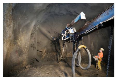
Spraying polymerenhanced concrete onto a tunnel wall in the Stetten salt mine. The sprayed concrete stabilizes the tunnel and keeps out water. The innovative formulation also reduces rebound during spraying, thus minimizing wastage and material consumption (photo: Wacker Chemie AG).
