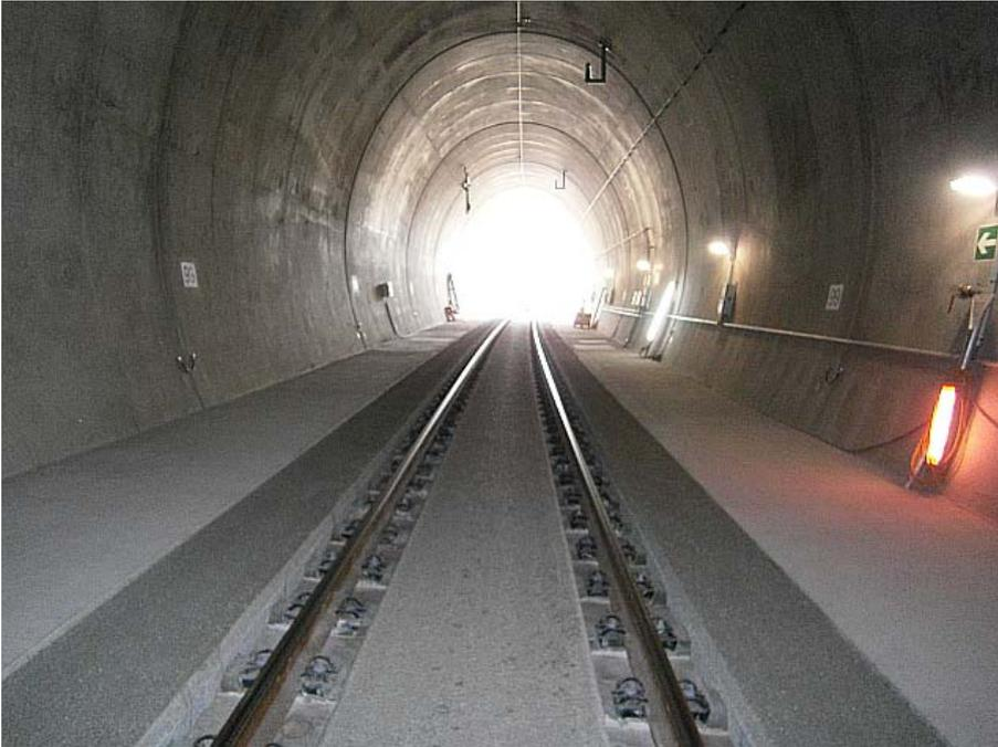
Drainage concrete modified with ETONIS<sup>®</sup> 260 is spread between and beside tracks and thus provides rescue vehicles and fire trucks with fast access to railroad tunnels. The new concrete is quick to put down, extremely durable and stable, and thus ideal for applications in road, tunnel and underground construction (photo: Wacker Chemie AG, courtesy of Deutsche Bahn AG).
