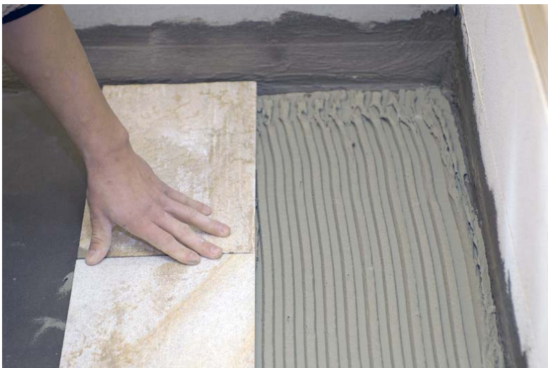
When applied under tile adhesives, sealing slurries modified with VINNAPAS® protect walls and floors against moisture in damp rooms, such as baths and basements (photo: Wacker Chemie AG).
