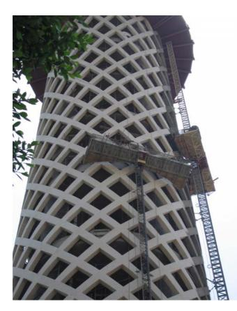
The extensive renovation of the Cairo Tower demanded the highest standards of quality for plaster, mortar, adhesive and grout additives. WACKER experts helped to develop formulations containing specialized VINNAPAS<sup>®</sup> polymer powders that now protect the television tower from heat, dryness and wind (photo: EKY).
