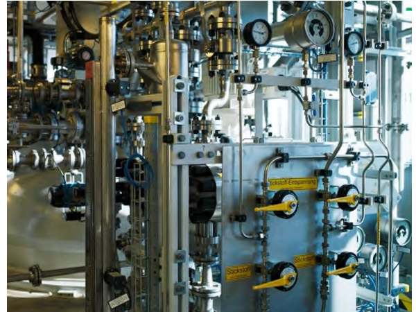
Reactor for producing dispersions in Burghausen (Germany)
