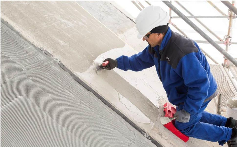
Application of VINNAPAS® 760 ED, a polymer dispersion that is ideal for flexible, two-component waterproofing membranes to create permanent, hard-wearing seals in water pipes, sewers and damp rooms such as kitchens and bathrooms.
