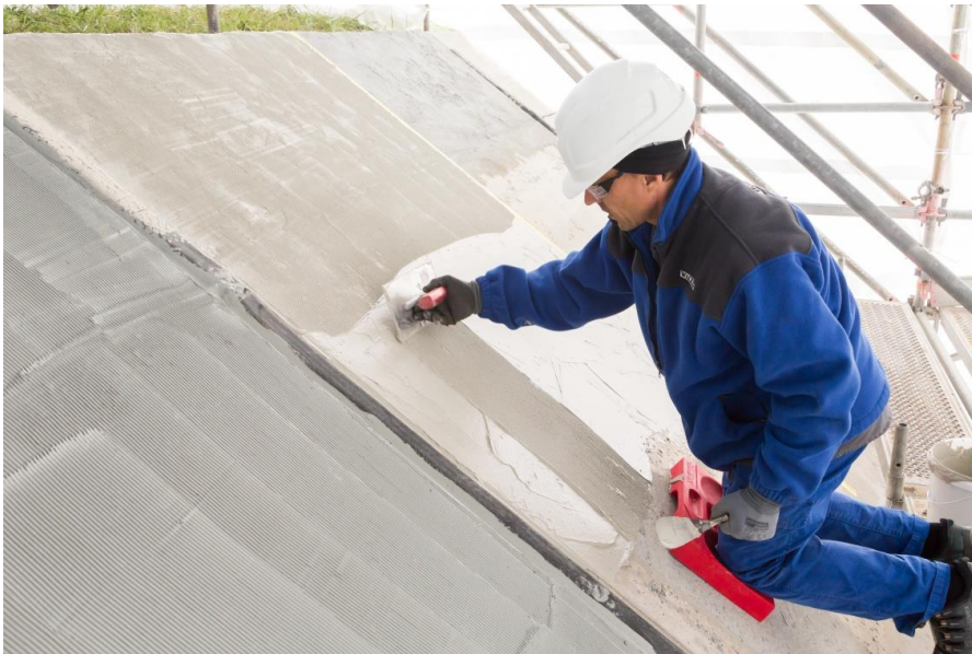
Outdoor weathering tests: The new VINNAPAS® 760 ED dispersion is ideal for flexible two-component sealing slurries for creating permanent, hard-wearing seals in damp rooms, such as kitchens and bathrooms, as well as for water pipes and sewers.
