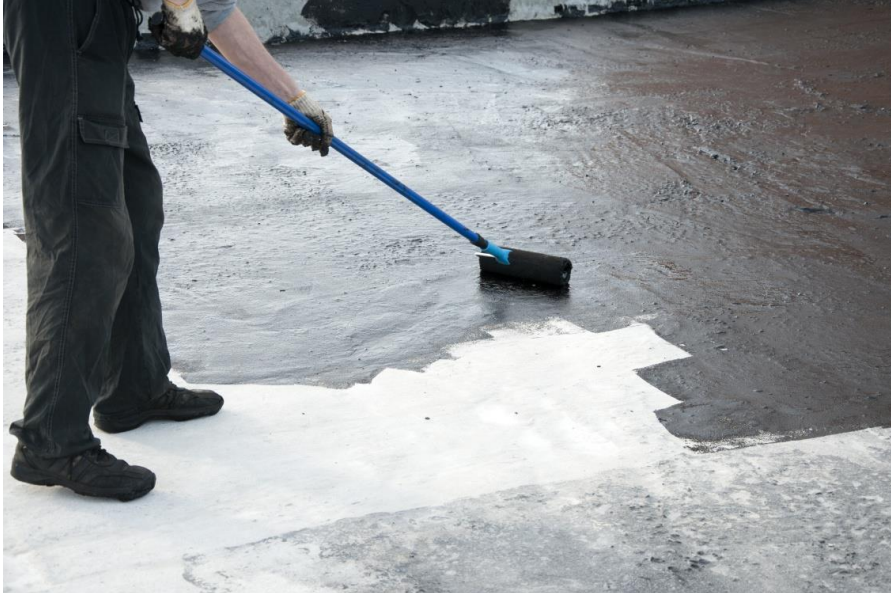
Coating a concrete surface with liquid bitumen
