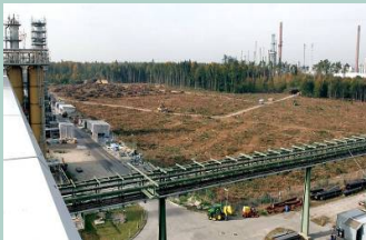
November 2006 Preparing the location
