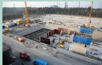
March 2007 Laying the foundations
