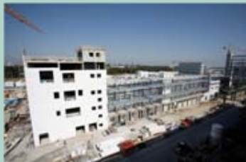
October 2007 New reactor hall
