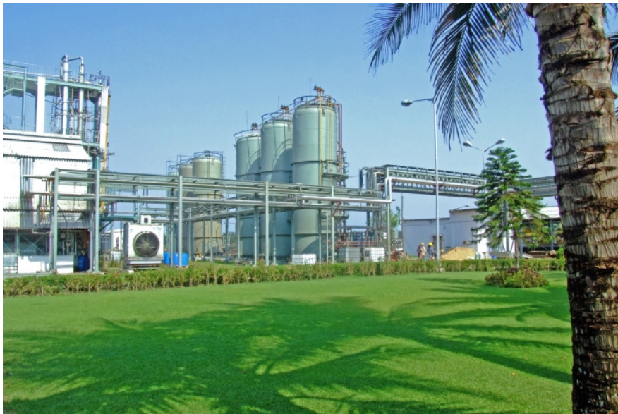
Wacker Metroark Chemicals’ production facility in Kolkata, India. The joint venture, in which WACKER has a 51 percent stake, produces silicones for the textile, personal-care, automotive, and construction sectors (photo: Wacker Chemie AG).
