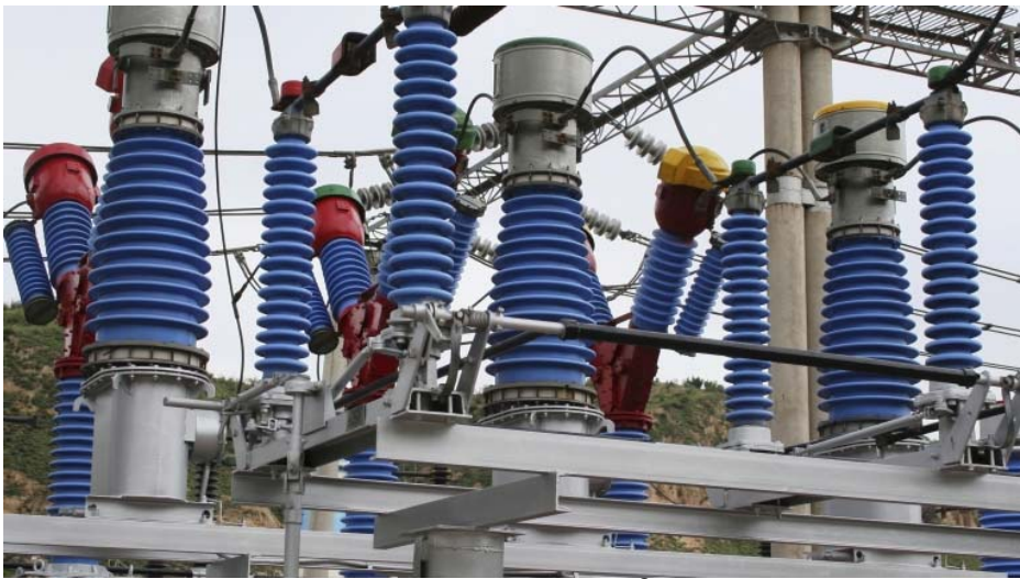
Porcelain insulators coated with POWERSIL®. Lab and endurance tests show that the hydrophobic properties of insulator coatings from WACKER SILICONES remain almost unaltered even after many years of weathering. (Photo: Wacker Chemie AG)
