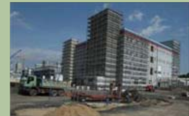
May 2010 Deposition reactor hall
