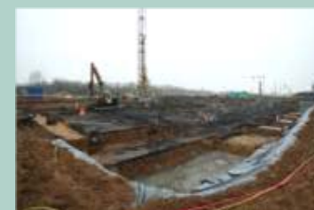
March 2009 Site preparation
