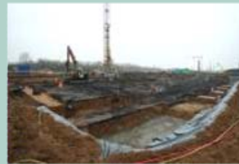
March 2009 Site preparation
