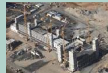
August 2009 Deposition reactor hall
