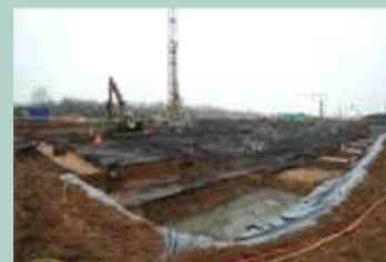
March 2009 Site preparation
