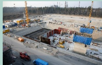
March 2007 Laying the foundations
