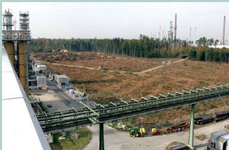
November 2006 Preparing the location
