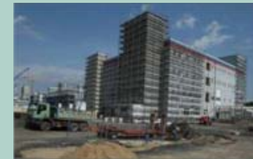
May 2010 Deposition reactor hall
