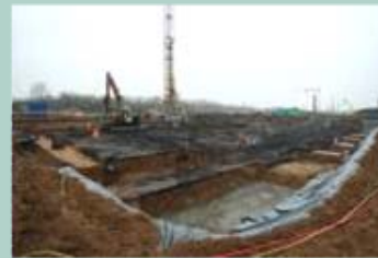
March 2009 Site preparation
