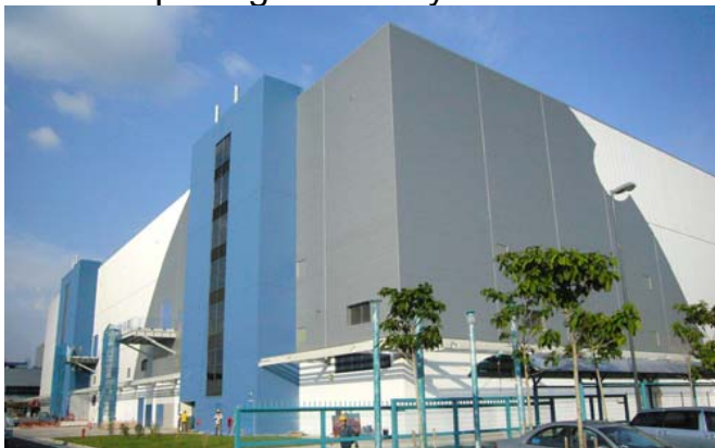
South west side view on fab building SSW
