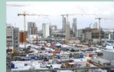
March 2010 View on construction site
