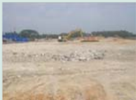
August 2006 Preparing the ground
