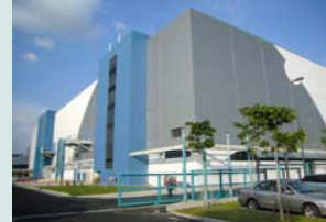
January 2008 Fab completed
