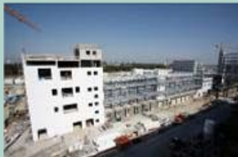
October 2007 New reactor hall
