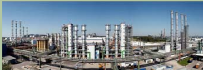
May 2010 Polysilicon production site
