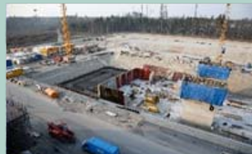
March 2007 Laying the foundations
