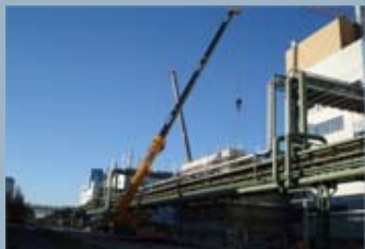
December 2006 Plant construction
