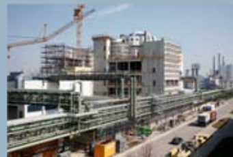
April 2007 All equipment in place
