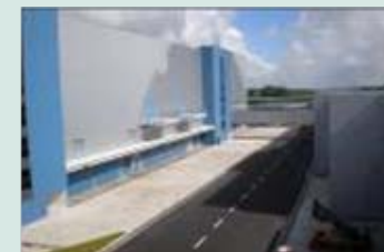
January 2008 Fab completed
