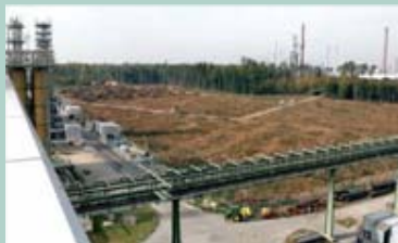
November 2006 Preparing the location
