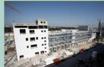
October 2007 New reactor hall
