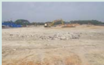
August 2006 Preparing the ground
