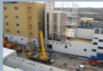
February 2007 Lifting in storage silos
